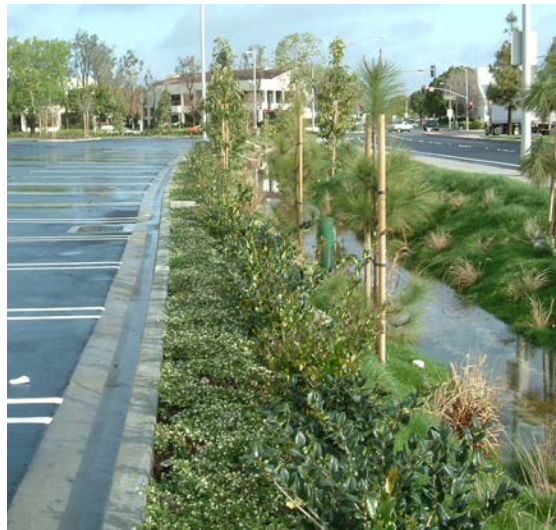
Bioswales and permeable paving allow stormwater runoff to percolate into the soil rather than flow directly into storm drains.
