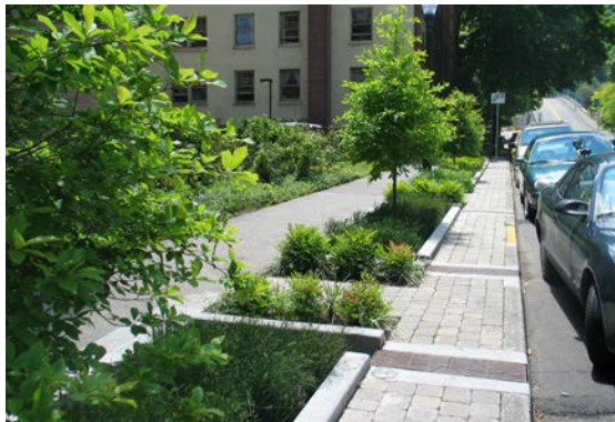
Filtration planter boxes with street trees help treat runoff.
