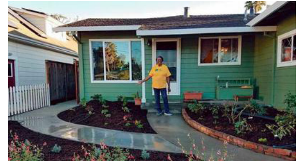
Accessory Dwelling Units can be built in backyards, as an addition, or even within an existing home.
