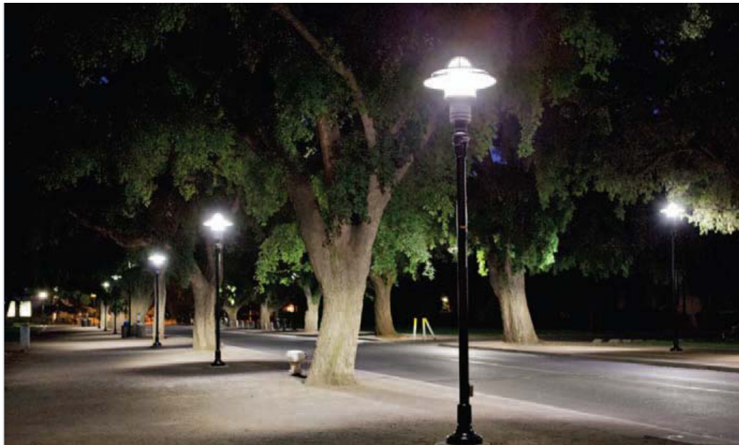
Improving lighting in public spaces is important to Alisal residents.
