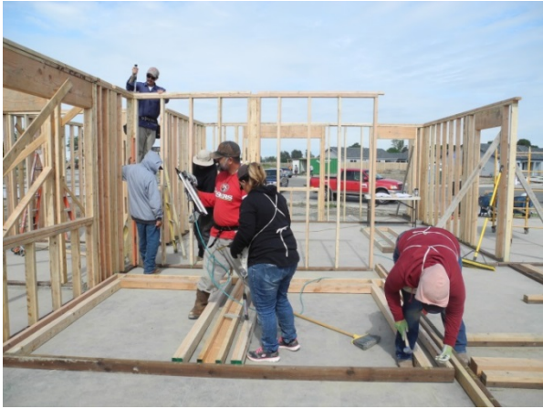
Building, Reedley Subdivision
