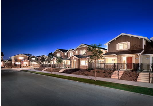
Azahar Apartments, Ventura 59 units, Opened 2012 Cabrillo Economic Development Corporation
