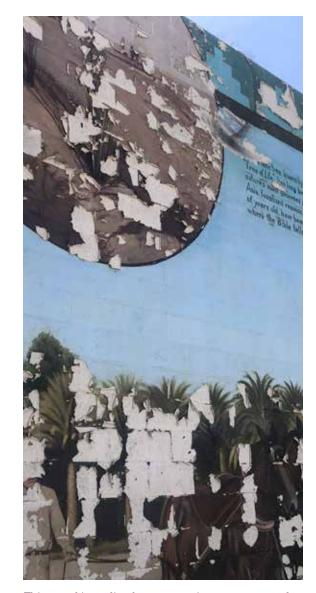
This mural is peeling because a primer was not used before applying exterior grade paint and sealant. The mural was restored by Evergreene Architectural Arts (Photo by Brooke Beare.)
