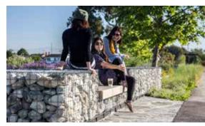
Gabion retaining and seat wall with integrated bench. (Photo by: SWA)
