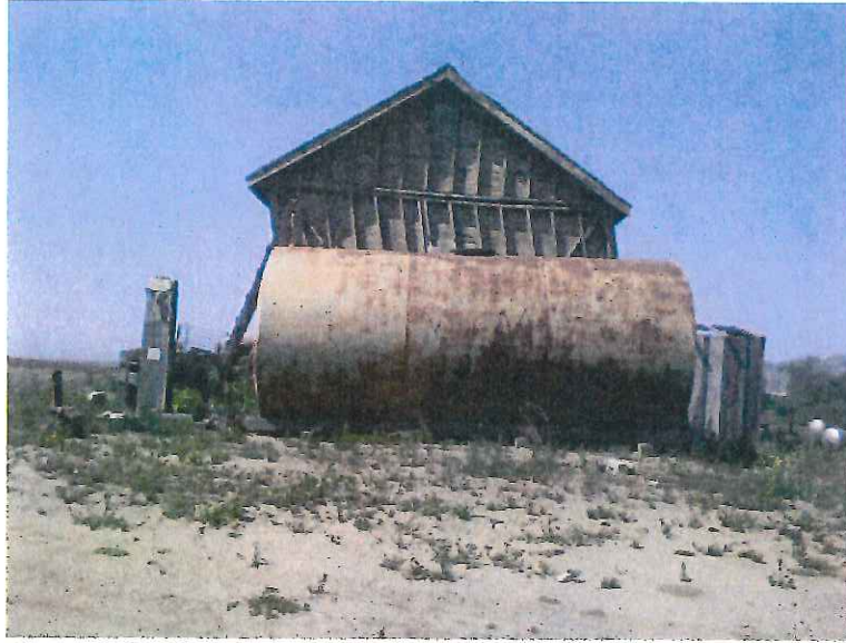
Photograph 3: Above ground gasoline storage Tank C.
