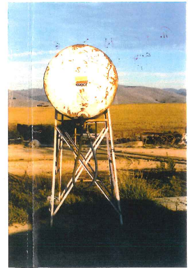
12. Parcel 7; Above-ground tank.
