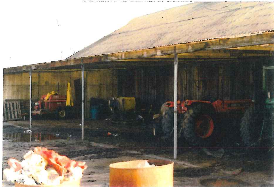
7. Parcel 4; View of side of barn.
