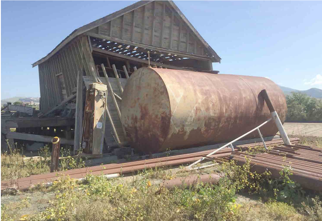
Photo No. 5 APN 153-091-001 – Abandoned fuel aboveground storage tank
