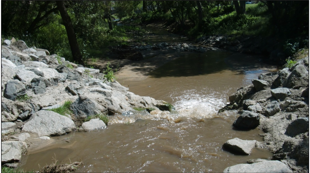
Figure 16 Concreted rip rap boulders control the channel gradient along Little River Drive.
