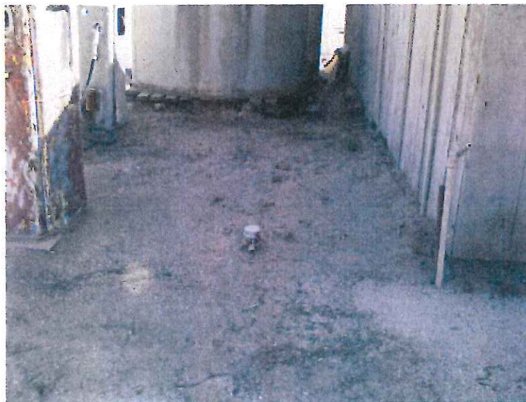
Photograph 2: View of fill pipe for underground storage tank.
