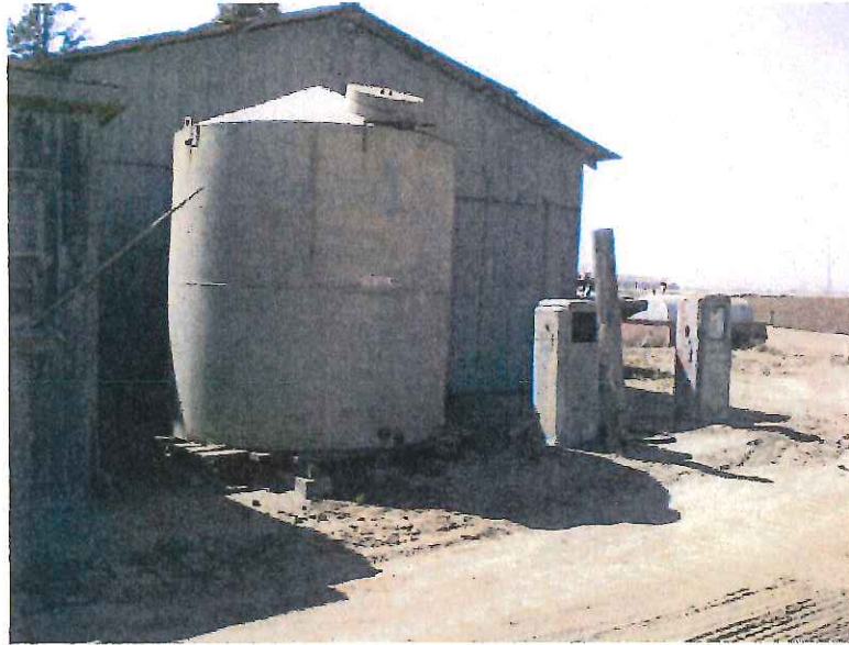
Photograph 1: Above ground diesel storage tanks (Tank A in foreground Tank B in right background of photograph).
