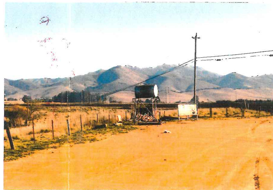
2. Parcel 6; Above-ground tank.
