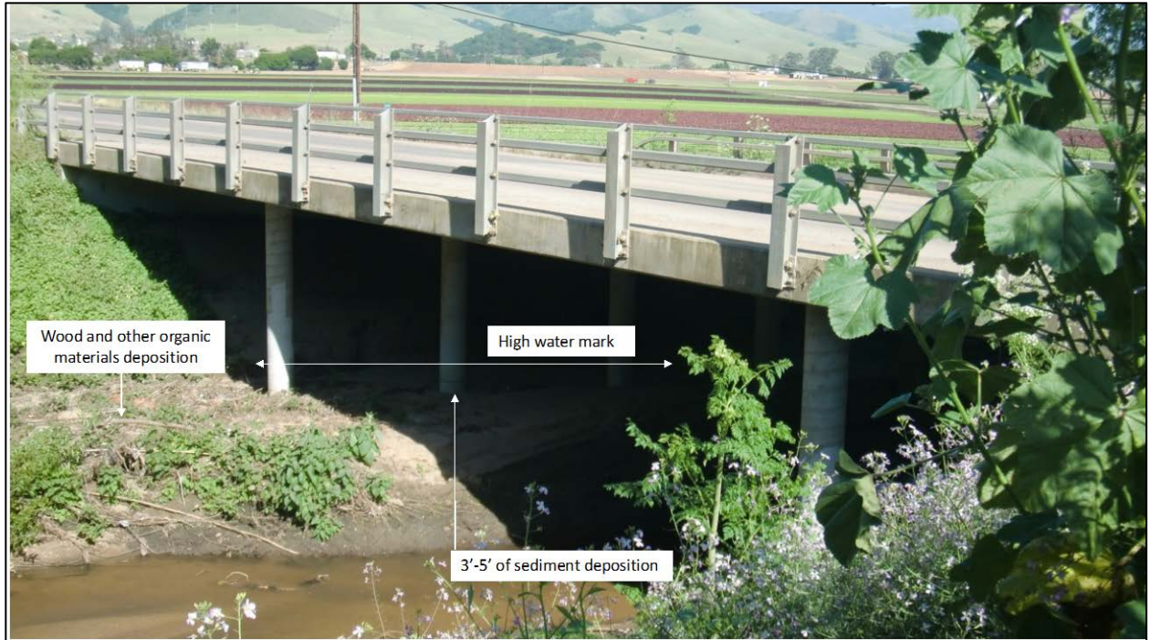
Figure 3 Gabilan Creek at bridge on Natividad Road with distinct indicators of high flow events experienced by the region in the 2016-2017 wet winter season. Downstream to the right.
