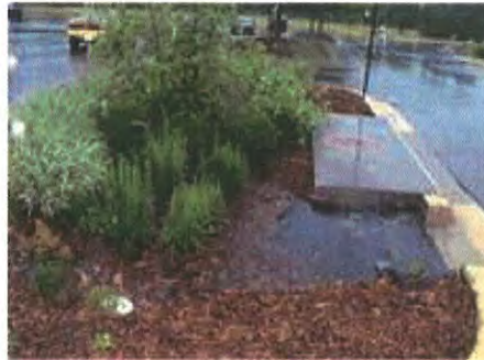
Figure 3-4039: Curb Opening Design for a Landscape Detention System Located Upstream of a Conventional Storm Drain Inlet (left photo) and a Bioretention System Retrofit into an Existing Parking Lot Island (right photo)
