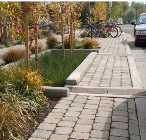
Pervious pavers used for street sidewalk
