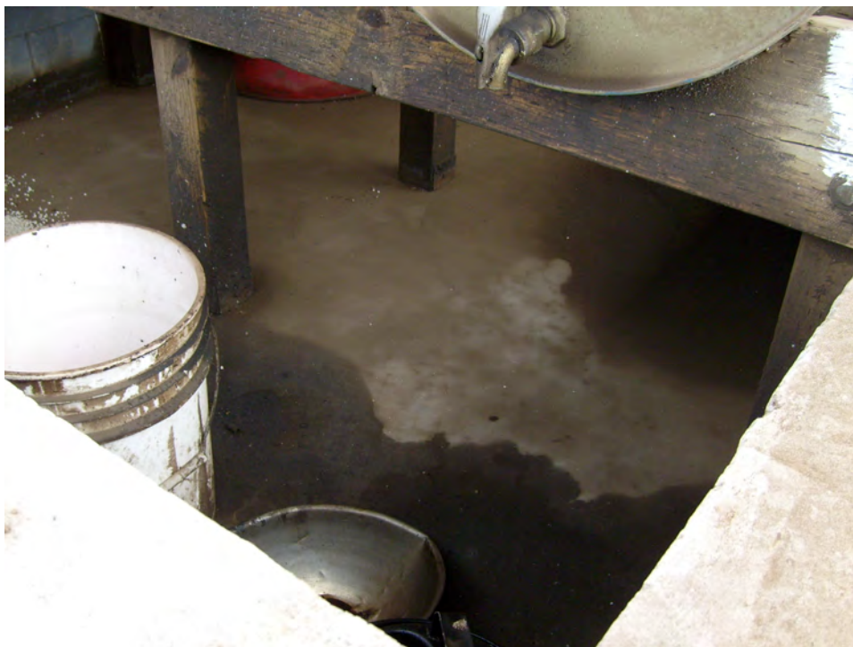
PHOTO 10: View of aboveground tank containment area floor at site
