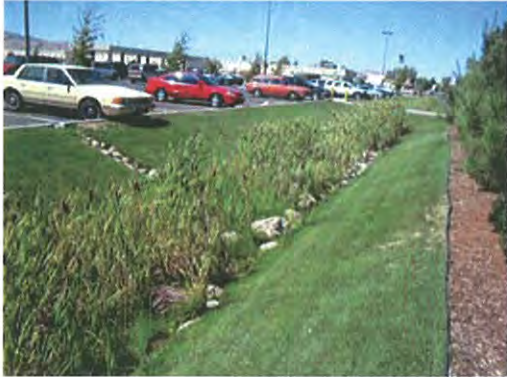
Figure 3-15: Parking Lot Bioretention
