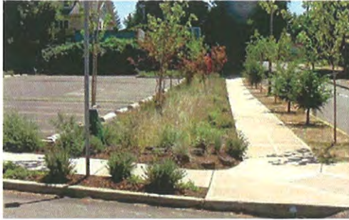
Figure 3-398: Landscape Detention Basins Located at the Edge of a Parking Lot (left photo) and in a Parking Lot Island with Turf and Shrubs and Trees (right photo)
