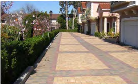
Figure 2-37: This residential driveway utilizes pervious joint pavers in San Mateo County.
