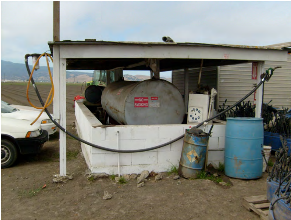
PHOTO 7: View of diesel tank at site
