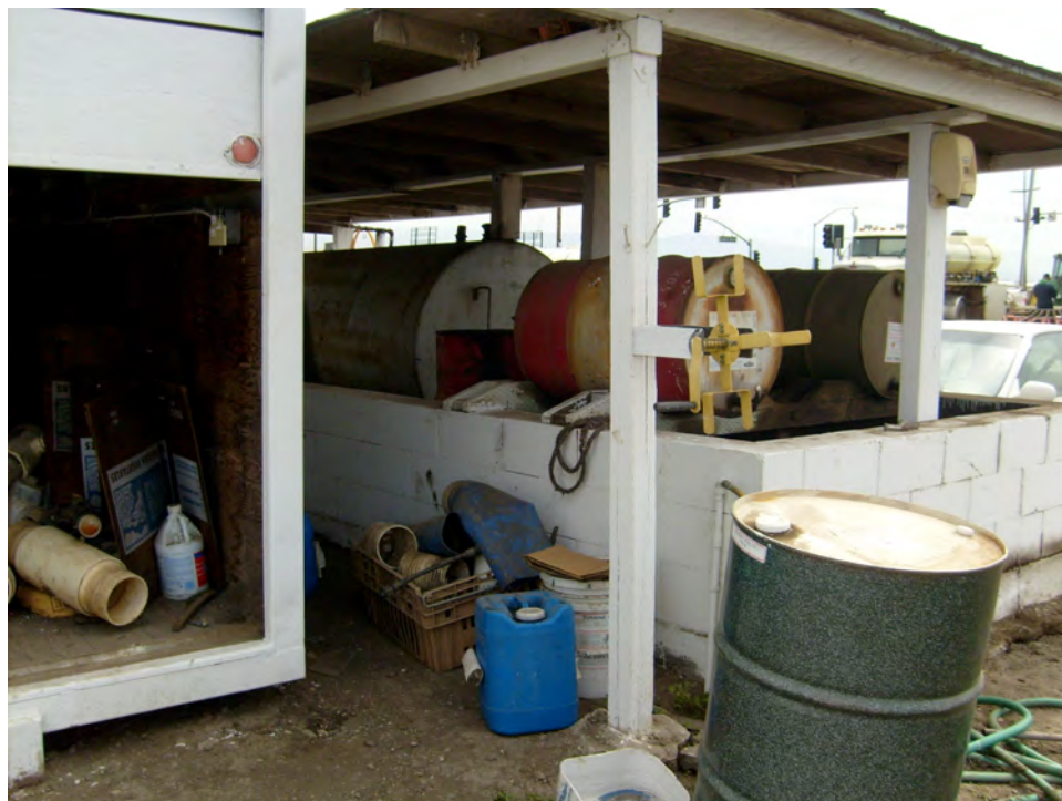
PHOTO 8: View of diesel tank, oil drums, and other materials at site
