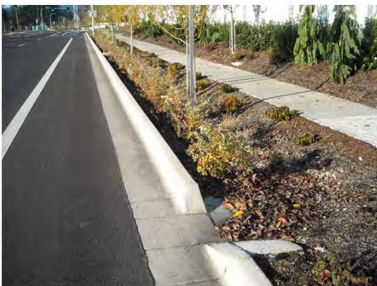
Figure 2-54: An arterial street with a vegetated swale.
