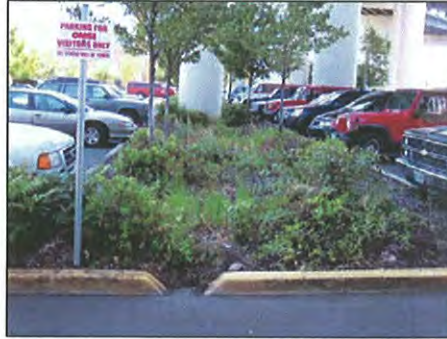
Figure 3-34: Parking Lot Island Bioretention System
