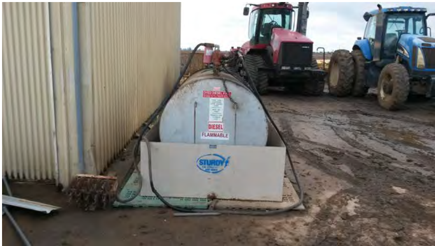
Photo 6 – APN 211-011-009 Approximate 500 gallons diesel fuel AST; view to the west.
