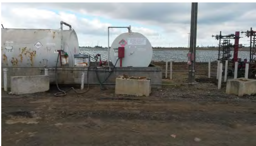
Photo 8 – APN 211-231-012 & -013 Approximately 1,000 gallon gasoline AST, view to the west.
