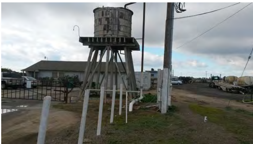
Photo 9 – APN 211-231-012 & -013 Wooden water tank and tower with residence in background; view to the west.
