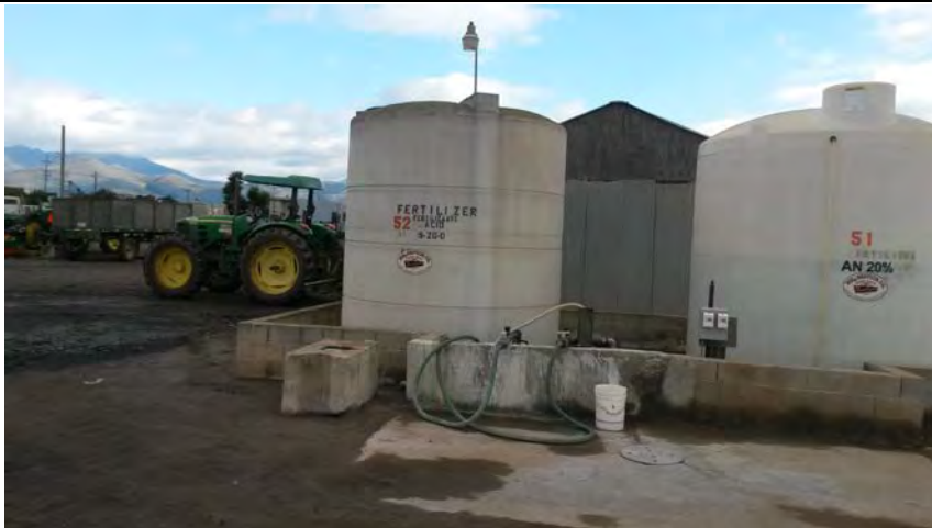
Photo 7 – APN 211-231-012 & -013 Approximately 3,000 gallon fertilizer storage tanks, view to the southeast.
