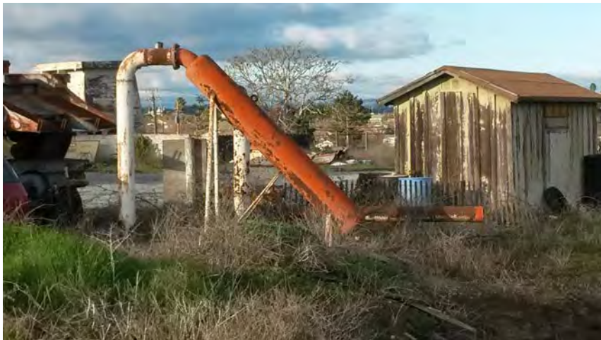
Photo 2 – APN 211-011-002 Drums next to shed; centrifugal sand separator (painted orange) and piping associated with an agricultural water supply well, view to the northwest.
