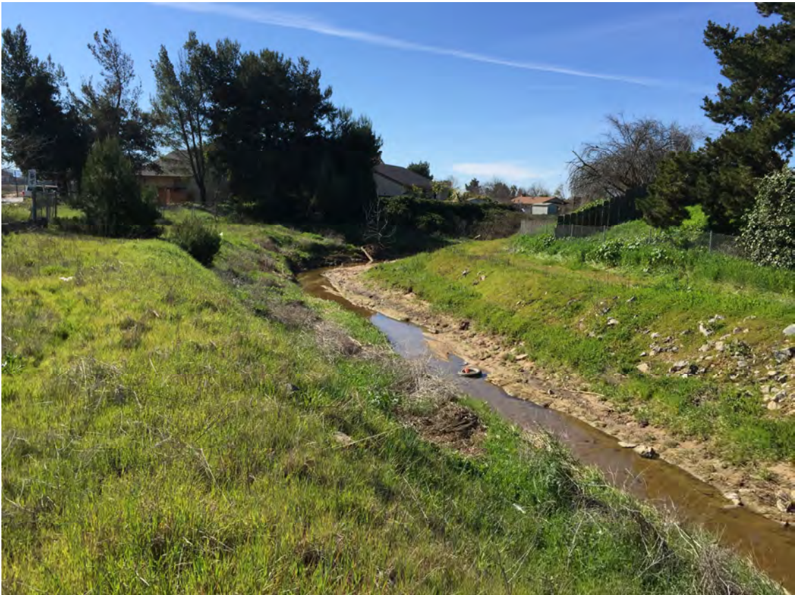
Plate 4- Santa Rita Creek looking south towards the point of the culvert discharge
