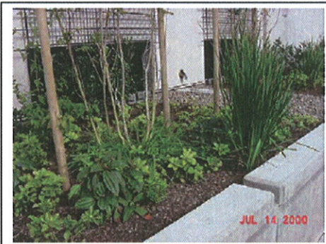
Figure 3-5049: Stormwater Planters Installed Next to Office Buildings (Source: Portland BES)
