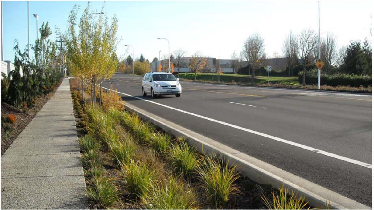
Figure 4-44: EXAMPLE: This arterial street utilizes a vegetated swale to accept stormwater from the street. This green street also uses sidewalks made from pervious concrete.
