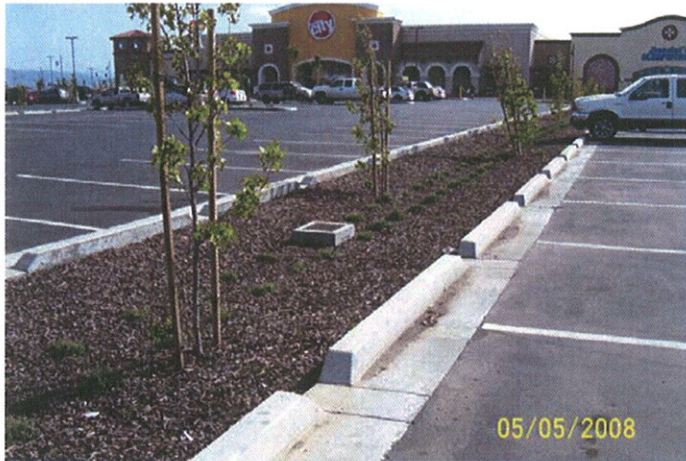
Figure 3-17: Curb Cuts Direct Water into a Parking Lot Bioretention System in the City of Salinas
