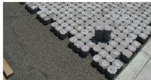
Figure 2-44: Sand-set interlocking concrete unit pavers create gaps between adjoining pavers and allow water to soak into the ground.
