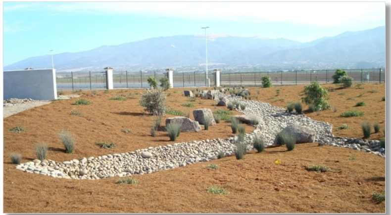
Example of a Post-Construction Stormwater BMP Facility
