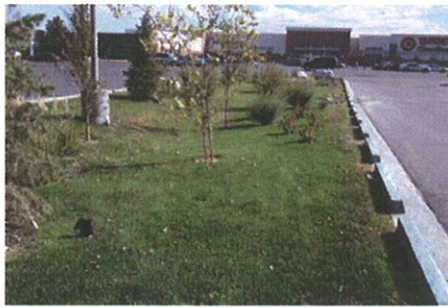
Figure 3-398: Landscape Detention Basins Located at the Edge of a Parking Lot (left photo) and in a Parking Lot Island with Turf and Shrubs and Trees (right photo)
