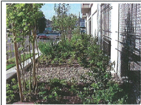
Figure 3-5049: Stormwater Planters Installed Next to Office Buildings (Source: Portland BES)
