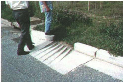
Figure 3-4039: Curb Opening Design for a Landscape Detention System Located Upstream of a Conventional Storm Drain Inlet (left photo) and a Bioretention System Retrofit into an Existing Parking Lot Island (right photo)
