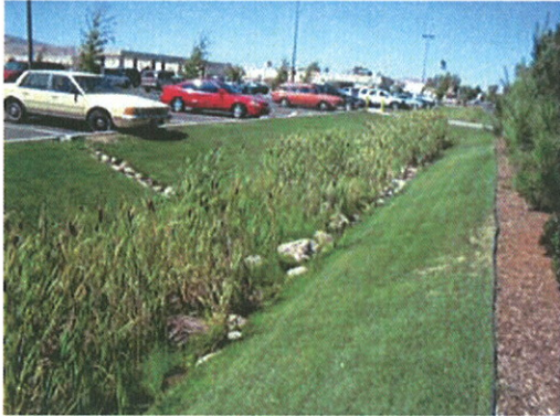
Figure 3-15: Parking Lot Bioretention
