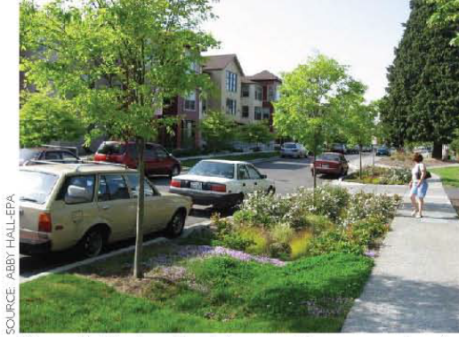
Figure 2-47: A residential street with a vegetated swale.
