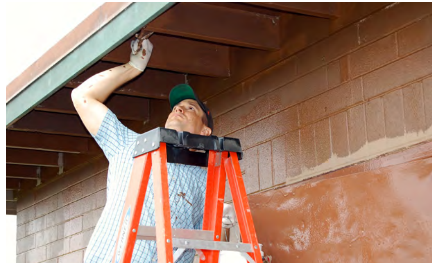
Restorations and upkeep help maintain existing assets
