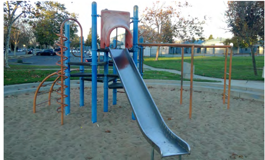
Several older playground structures were noted for replacement
