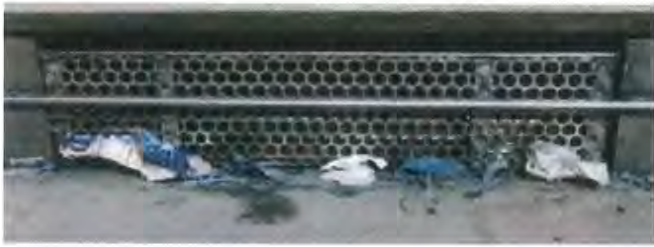
AUTOMATIC RETRACTABLE INLET SCREEN – ONE PIECE
