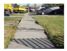
These sidewalk upheavals create problems for pedestrians as demonstrated by the following table that shows claims for trips and falls in City sidewalks. These claims represent reported injuries caused primarily by sidewalks damaged by tree roots. There is no measure of the unreported incidents due to falls caused by deficiencies in the sidewalk system. As the data
