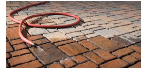
Permeable Pavers on Permeable Material
