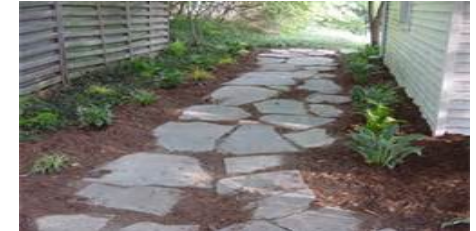
Open Stone Paving On/Draining to Permeable Areas
