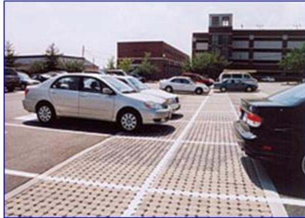
**Figure 1: Example of an Open Jointed Block Paver installation**
