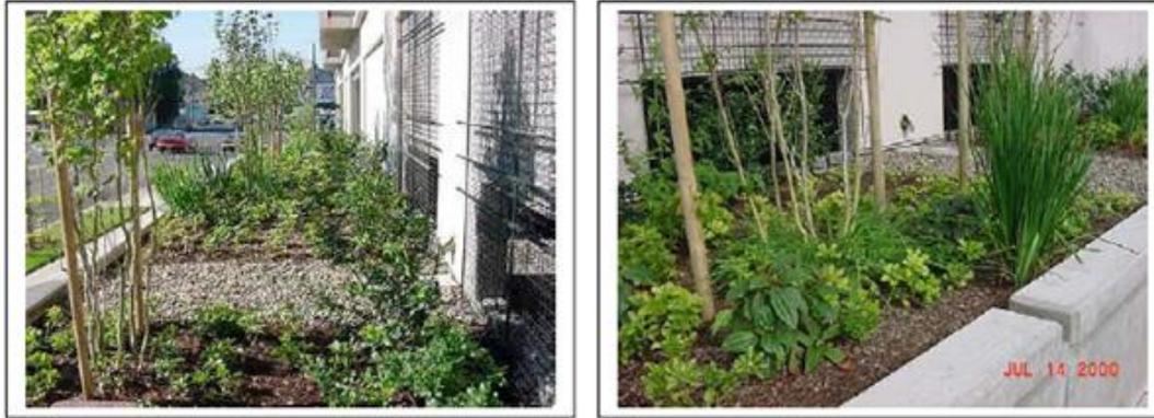
**Figure 2: Stormwater Planters installed next to office buildings** (Source: Portland BES)
