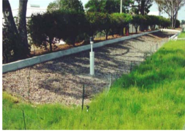
Figure 2: Infiltration Trench (Source: LA LID Manual)
