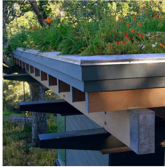
Figure 9: Green roof on Carmel Valley, CA Residence (Photo: Jonathan Feldman Architecture)
