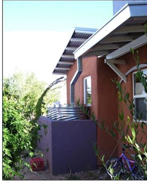
Figure 8: A rainwater capture and reuse system on a residential home. (Photo: Kennedy/Jenks Consultants)
