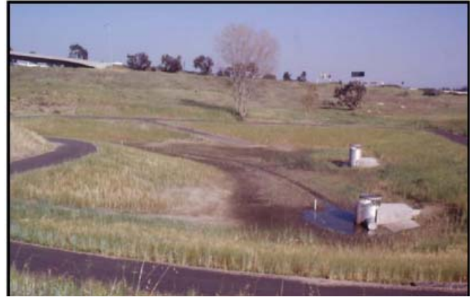
Figure 1: Infiltration Basin (Source: CASQA Stormwater BMP Handbook)
