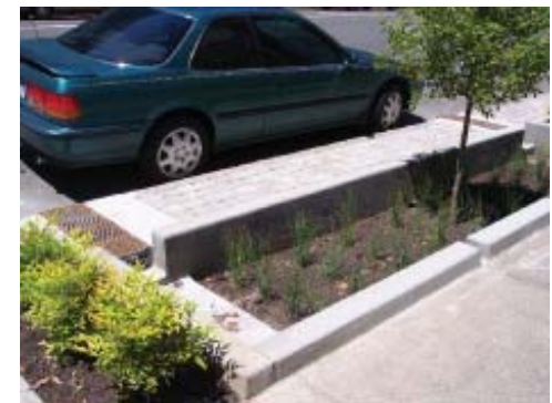
Bioretention basin along an urban roadway
